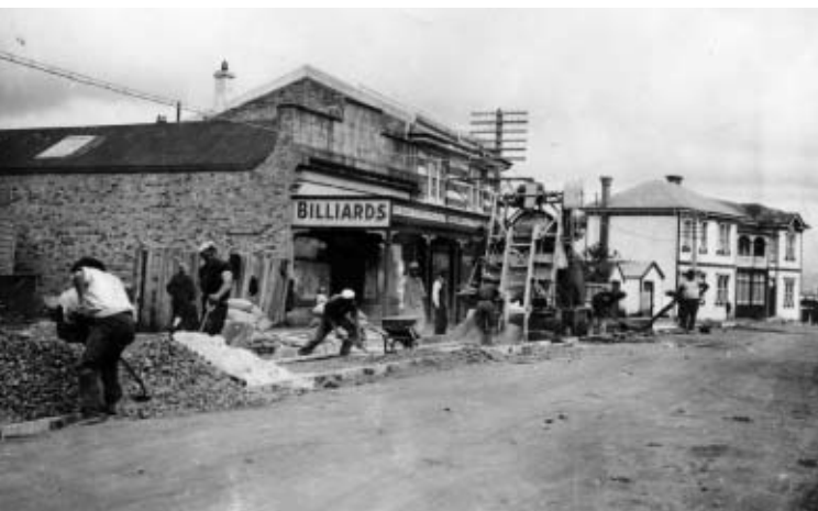
Laying concrete road, Queen St late 1920s. Northcote library collection.
